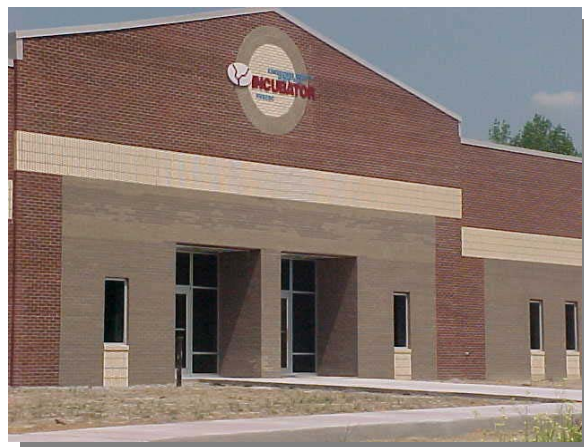
One of the RMECDC's most recent economic development initiatives, the Business Incubator facility, currently under construction
