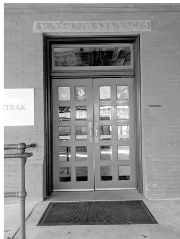
CLEAN AND PAINT ALL EXISTING EXTERIOR DOORS AND GLASS. PAINT DOOR TO MATCH EXISTING COLOR. VERIFY IN FIELD.
