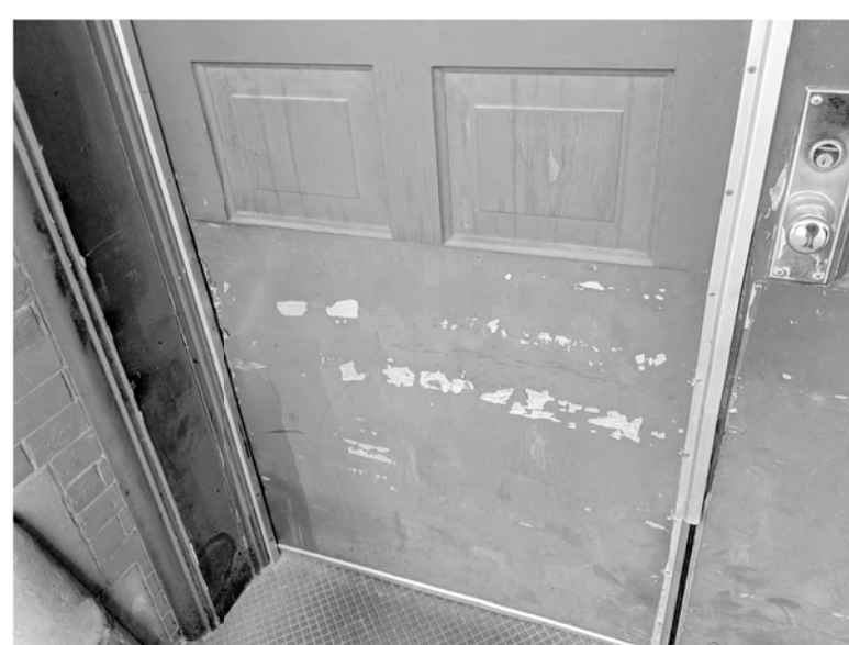
INSTALL NEW DIAMOND PLATE SHEETS TO EXISTING DOOR. SEE SPECIFICATIONS FOR SIZE AND COLOR. ③
