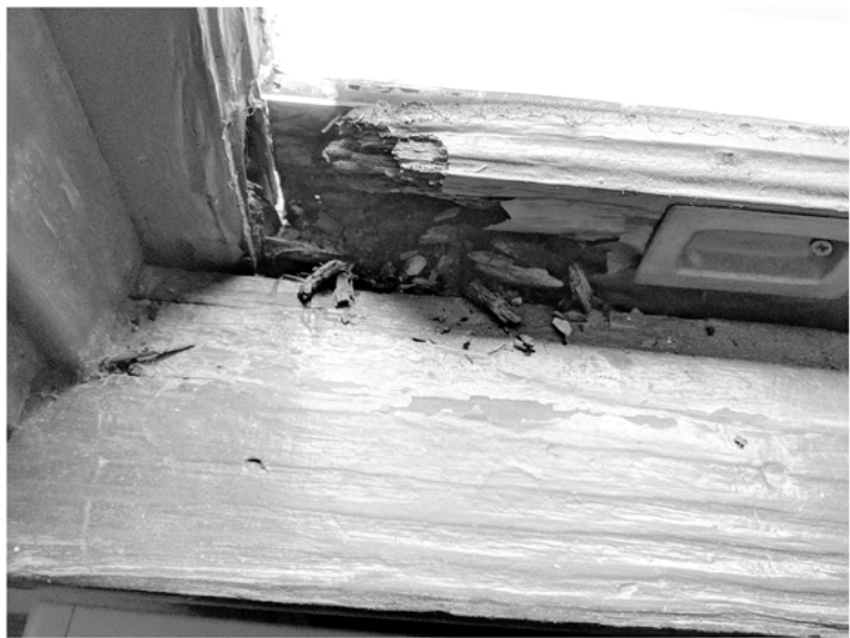
REPLACE EXISTING DAMAGED/ROTTEN WINDOW SILLS. PAINT TO MATCH EXISTING COLOR.
