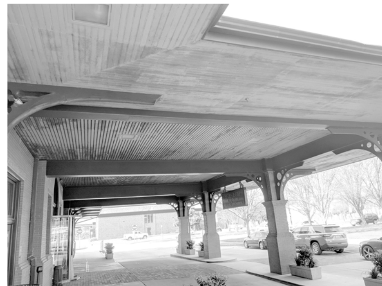
CLEAN AND PAINT EXISTING CANOPY UNDERSIDE, AND ROOF SOFFIT. APPROXIMATELY 11,200 SQUARE FEET COMBINED. COLOR TO MATCH EXISTING.
