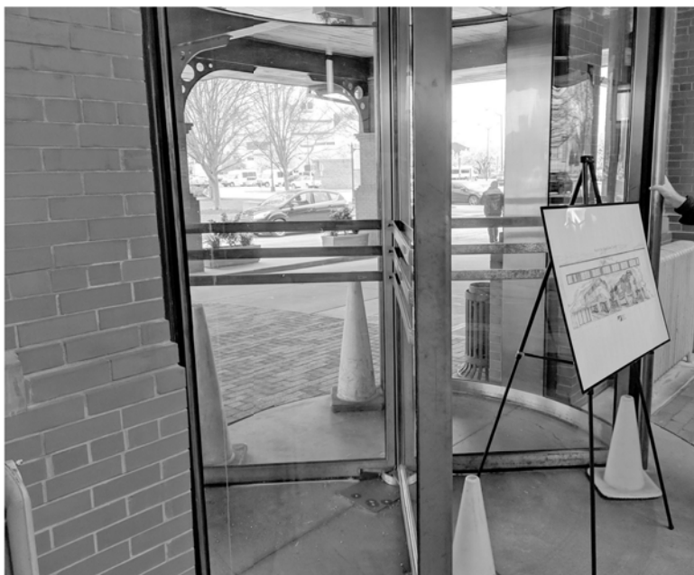
CLEAN REVOLVING DOOR. REPAIR HARDWARE. SEE SPECIFICATIONS.
