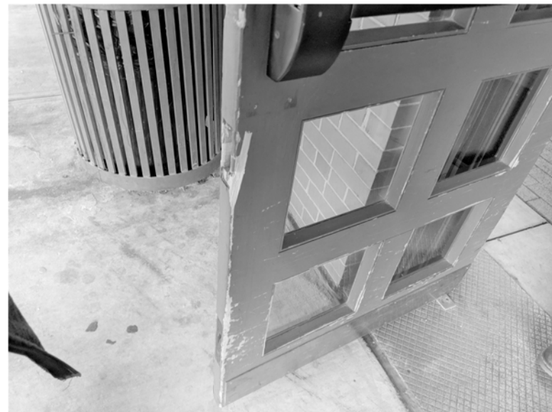
PATCH AND REPAIR ALL DAMAGED DOORS. ⑤
