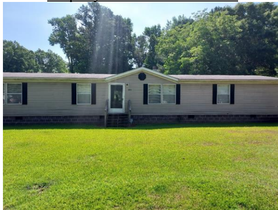
Property A: 301 Second Street
