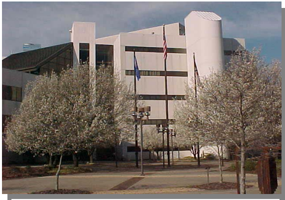
Rocky Mount City Hall Complex. Opened October 1982.
