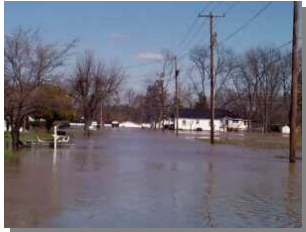
Damage from the flood wrought by Hurricanes Dennis and Floyd in 1999.
